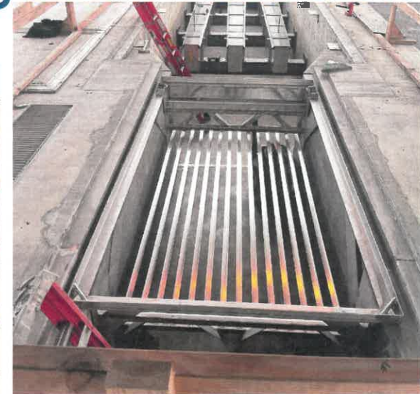
Adding new light bank and weirs
